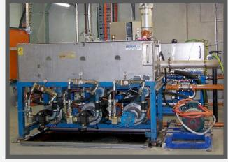
A new power unit was commissioned in a dedicated plant room. Existing pipework had to be tapped into. The old power unit was then disconnected and re-located to the plant room alongside the new unit. A 5" stainless steel balance pipe was installed between the two.
