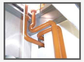
Additional pipework to the rooftop was required to allow the incorporation of the bank of heat exchangers.
