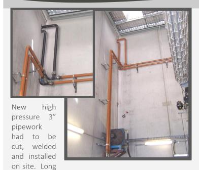
lengths had to be accurately measured, joined and secured along walls, floors and through sections of roof. Much of this involved working at heights (9-10m) and long runs (up to 18m). All pipes needed to be painted in a standard colour-coded protective coating.
