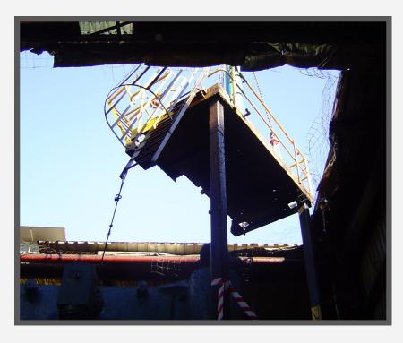
The main press body was lifted through the roof of the building using a 300 tonne crane before being reconditioned, repositioned and recommissioned.
