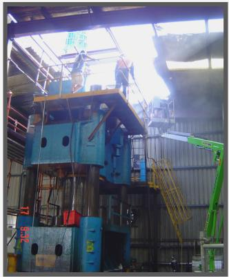
connection of the electrical equipment. The 3000 litre reservoir had to be emptied, cleaned, repainted and re-sealed. Special tools had to be manufactured. The eight nuts on the corner posts each weighed 300 kg and were difficult to remove after many years without being disturbed. All pumps, valves, tubework and hoses were carefully removed, tagged and notated. Every hydraulic and mechanical component was either overhauled or replaced.
